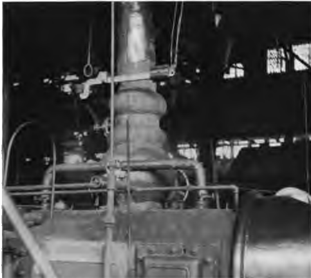
Fig. 3. Butterfly Valve with Counterweight and Trip Cords.*
